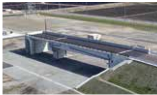
8 Bridge for testing
