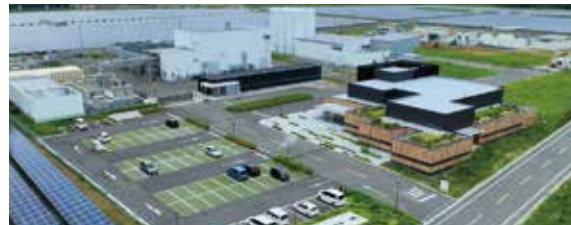
Fukushima Hydrogen Energy Research Field (Source: NEDO)
