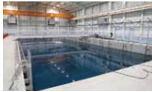
5 Indoor water pool testing building
