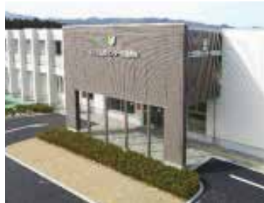
Medical & nursing care facility Futaba Medical Center (Tomioka Town)
